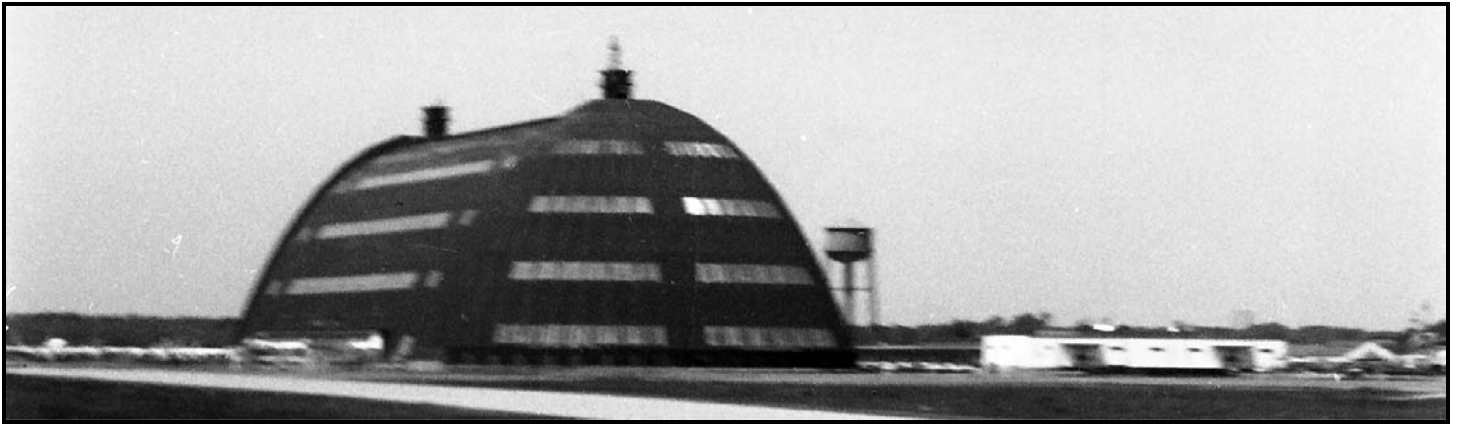
ABOVE: John Donatello provided this photograph of the old blimp hangar at NAS South Weymouth that was taken sometime during the early 1960s while he was with VP-912. This all-steel structure was called Hangar One or "The Big Hangar". It was one of two blimp hangars built on the base during the Second World War. The other blimp hangar, Hangar Two, was made primarily of prefabricated wooden components. It was located on the site of the base's modern-day CGA facility and control tower and was demolished during 1951 or 1952 to clear the way for runway construction. BELOW: Bob Kowalewski sent us this shot of VP-92's CAC-1 posed out on the ramp at NAS South Weymouth sometime during in the early to mid 1990s. Bob Mandeville's beard (far right) has been a no-no in the Navy for many years.
